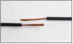
1. Strip wires 1/2" to 3/4" and lay opposing as shown. Slide sleeve over one wire.
